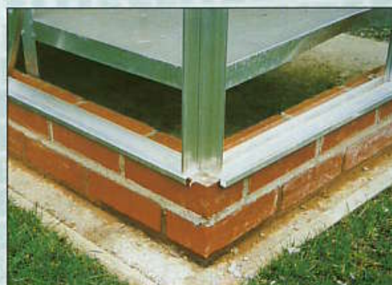
Overlapping cills demonstrate need for accuracy when building brick bases
